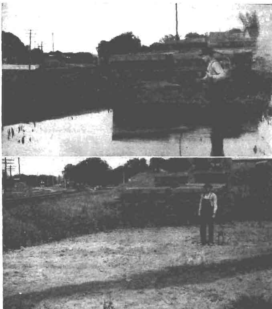
FIG. 85. Upper figure shows a pond adjacent to a railroad and caused by obstructing the natural drainage, a source of many mosquitoes every year. Larviciding, while serving the purpose of mosquito control, requires repeated expenditure of time, labor, and money. The lower figure shows the same spot after it had been permanently corrected by the railroad company.
